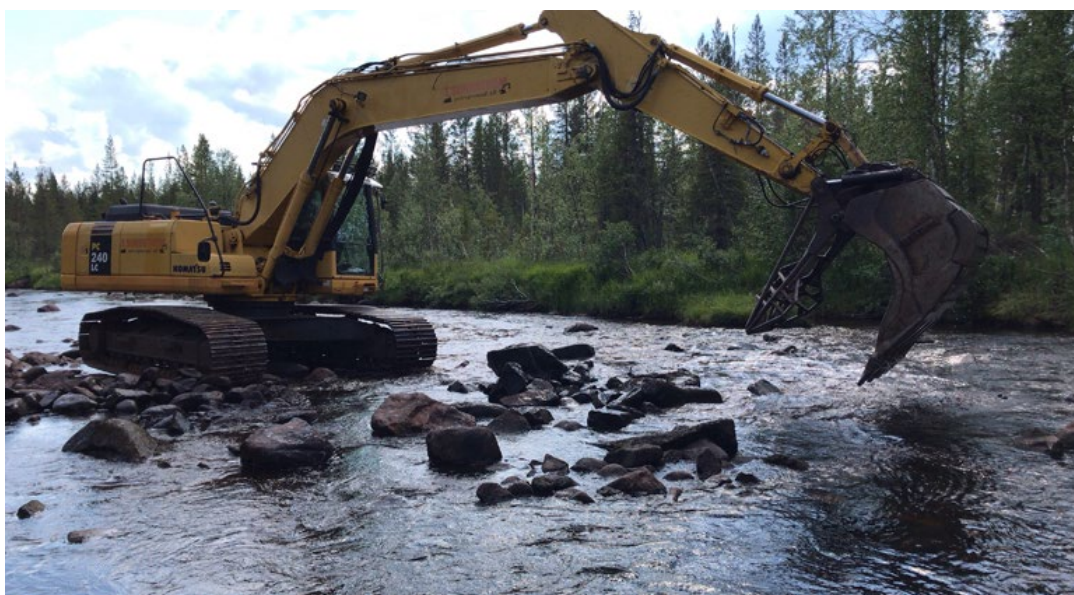
EMRA, Restoration in Pärlälven
